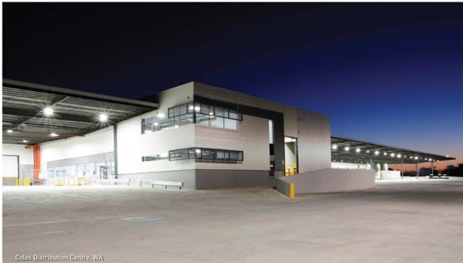
Coles Distribution Centre, WA
