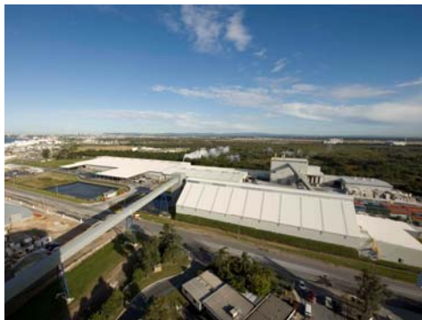
Pinkenba PLASTERBOARD plant, QLD
