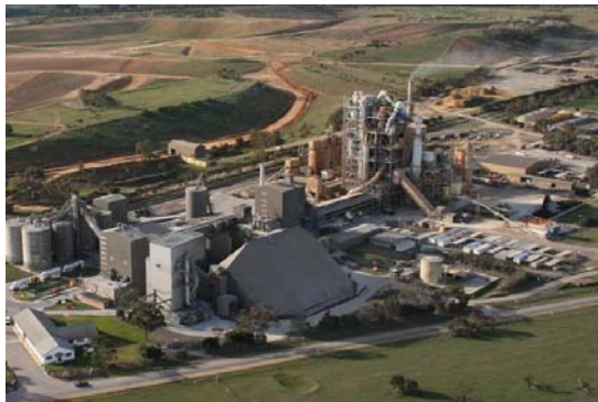
Blue Circle's Waurn Ponds CEMENT works
