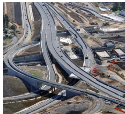
ASPHALT for the SAFELink project QLD
