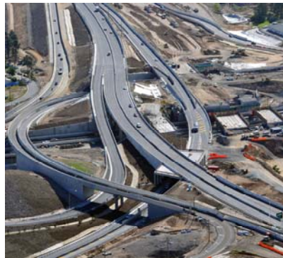
ASPHALT for the SAFELink project QLD
