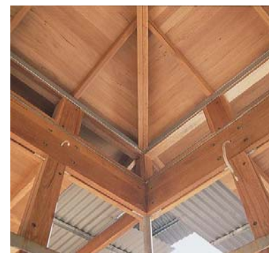
Hardwood TIMBER, roofing frame
