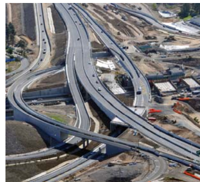
ASPHALT for the SAFELink project QLD
