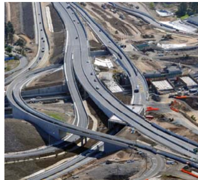
ASPHALT for the SAFELink project QLD
