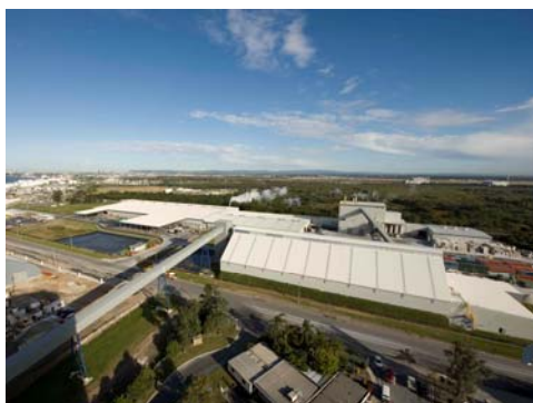
Pinkenba PLASTERBOARD plant, QLD
