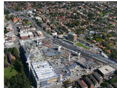
CONCRETE PLACING, Shopping Centre NSW
