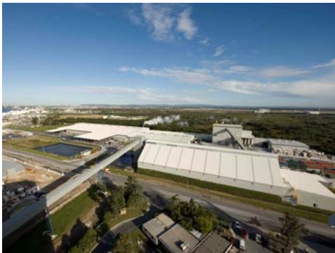
Pinkenba PLASTERBOARD plant, QLD
