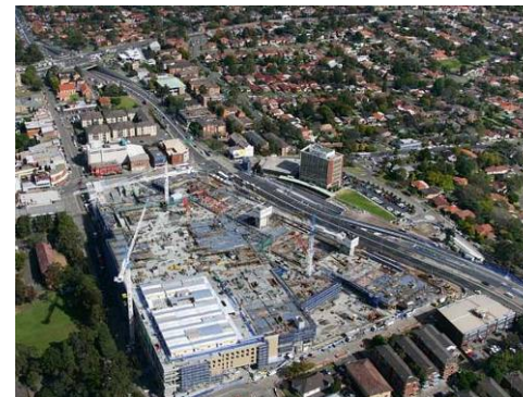
CONCRETE PLACING, Shopping Centre NSW
