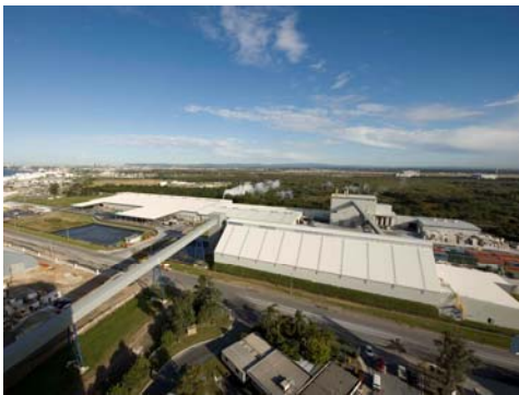
Pinkenba PLASTERBOARD plant, QLD
