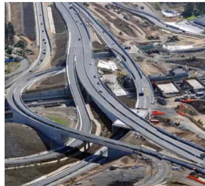
ASPHALT for the SAFELink project QLD
