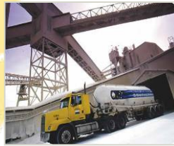
Blue Circle Southern Cement
