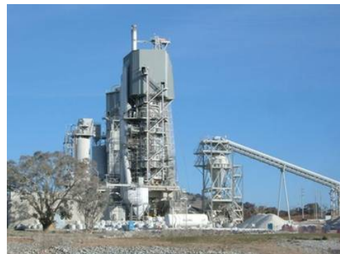
Galong LIME kiln re-started in December
