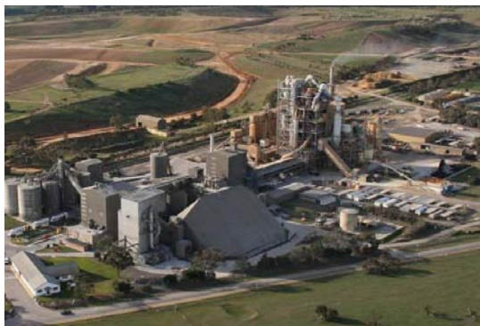
Blue Circle's Waurn Ponds CEMENT works
