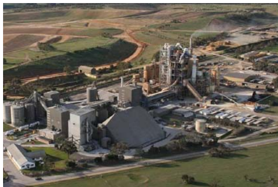
Blue Circle's Waurn Ponds CEMENT works
