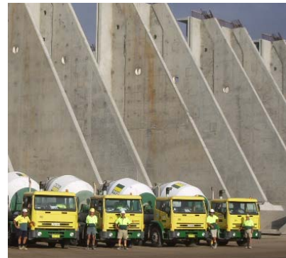
CONCRETE for the Port Botany Redevelopment NSW
