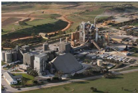
Blue Circle's Waurn Ponds CEMENT works
