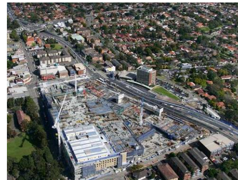
CONCRETE PLACING, Shopping Centre NSW
