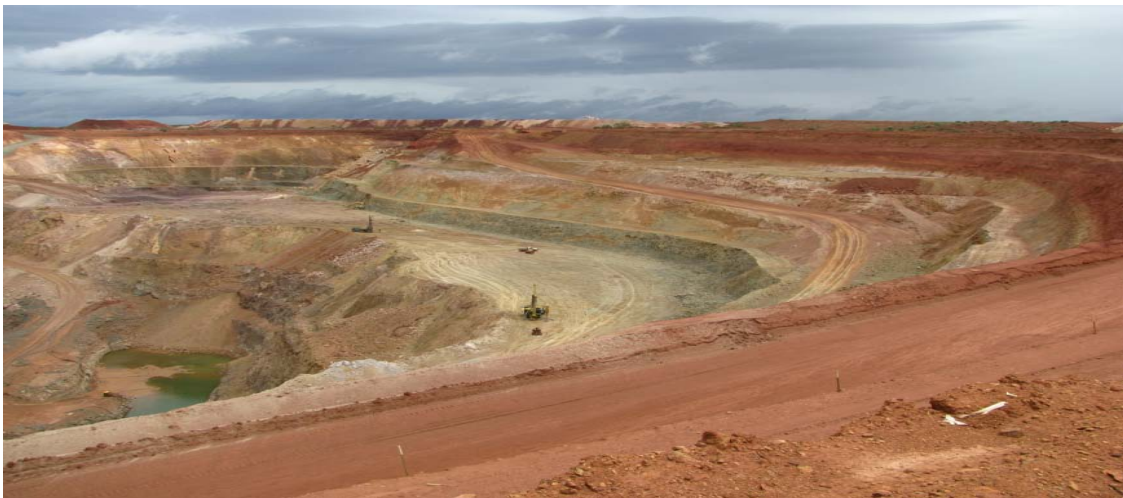
Photo 2: View of western cutback looking to the south.
